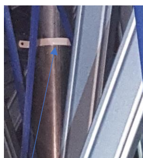
Flue through roof was correct
