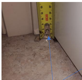
Approx. 4 mm difference across doors measured
